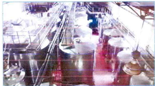
Wine Fermentation Tanks
